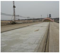
Fin rubber dam: The cross-section of fin rubber dam looks like a book with smooth appearance. The fin erects when inflated to form a rising angle to raise the water head during a certain overflow, and eliminate vacuum underneath the dam with certain depth of flow water, thus reducing the vibration and wearing out of the rubber bladder.
